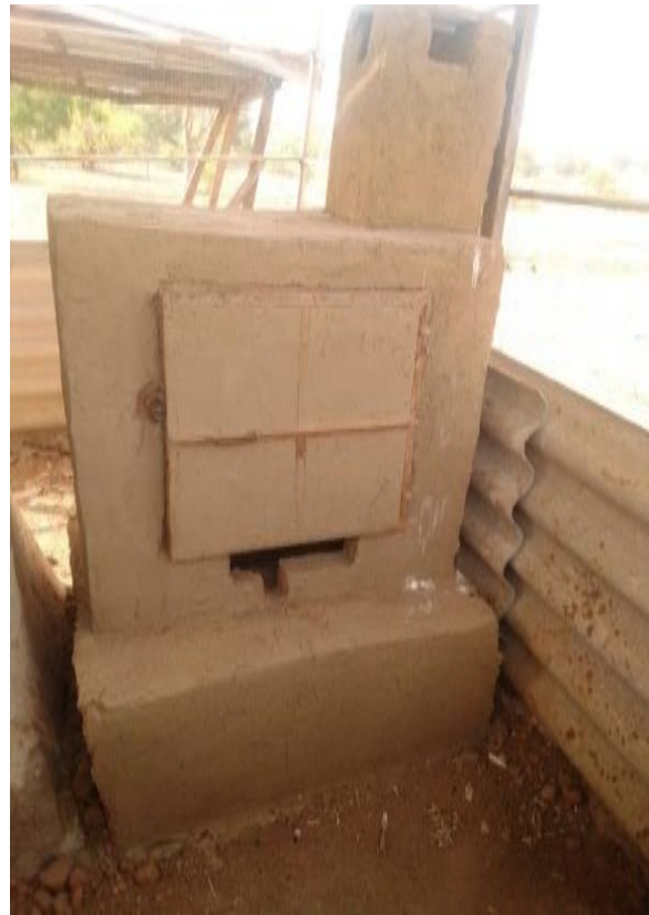
Plate 4; Plate 4; Kiln structure
