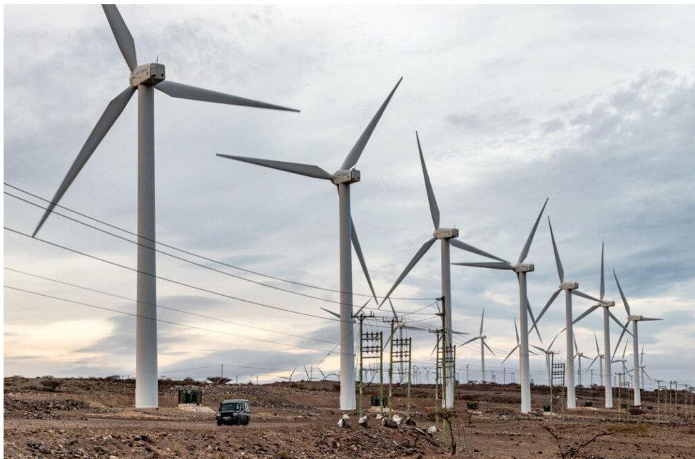
Figure 7: The 310 MW Lake Turkana Wind Energy Project in Kenya [25].
