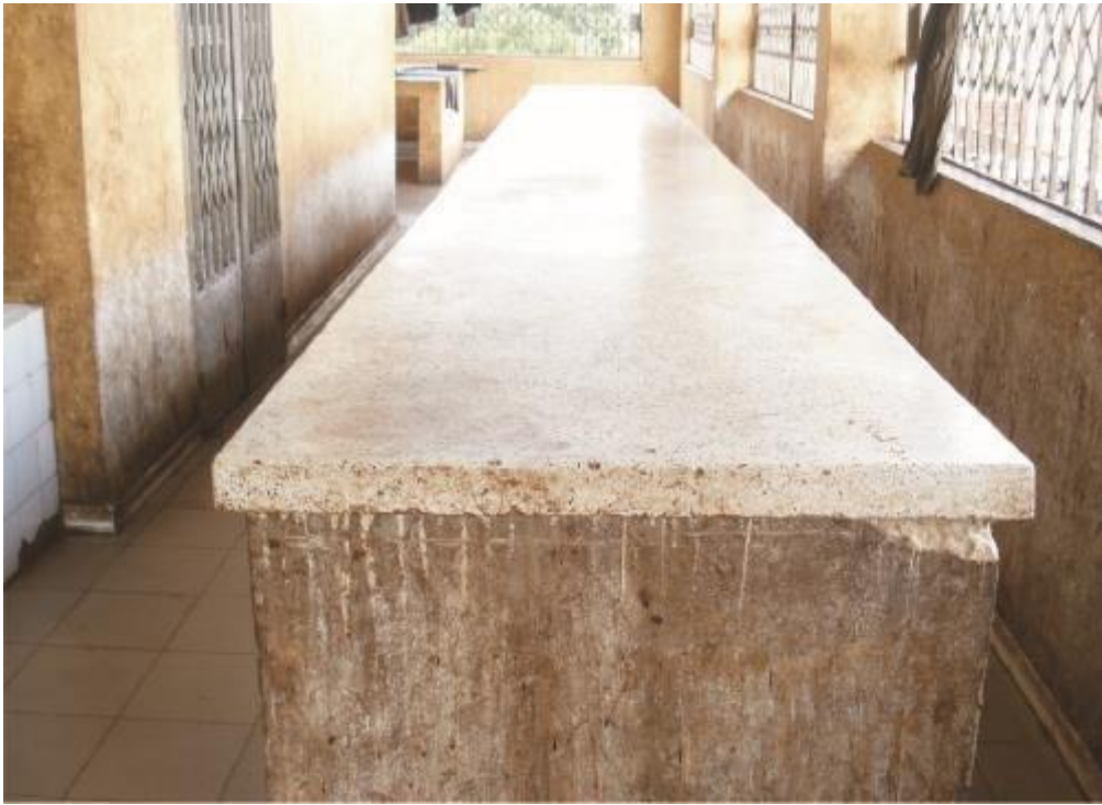
Fig 15: A marble top table for slaughter and processing of poultry, easy to wash and disinfect (produced in Mali)
